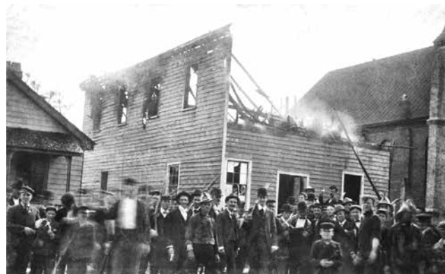
The remains of the office of the Black-owned newspaper The Daily Record after it was burned in the Wilmington coup and massacre, November 10, 1898.
